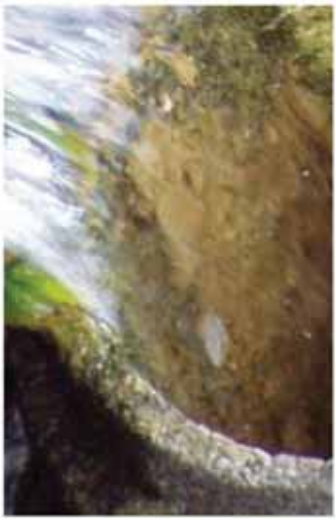
Answer: Wastewater pipe
